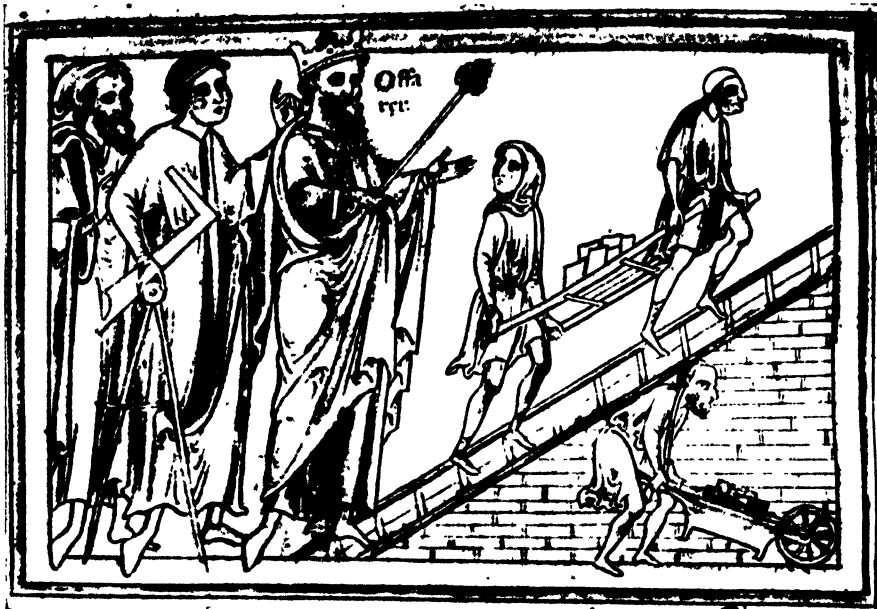
136. The King and his architect (with compass and ruler) visiting the building site of a cathedral (King Offa at St. Albans) . From an English manuscript of the Life of St. Alban probably painted by MATTHEW PARIS about 1260. Dublin, Trinity College
